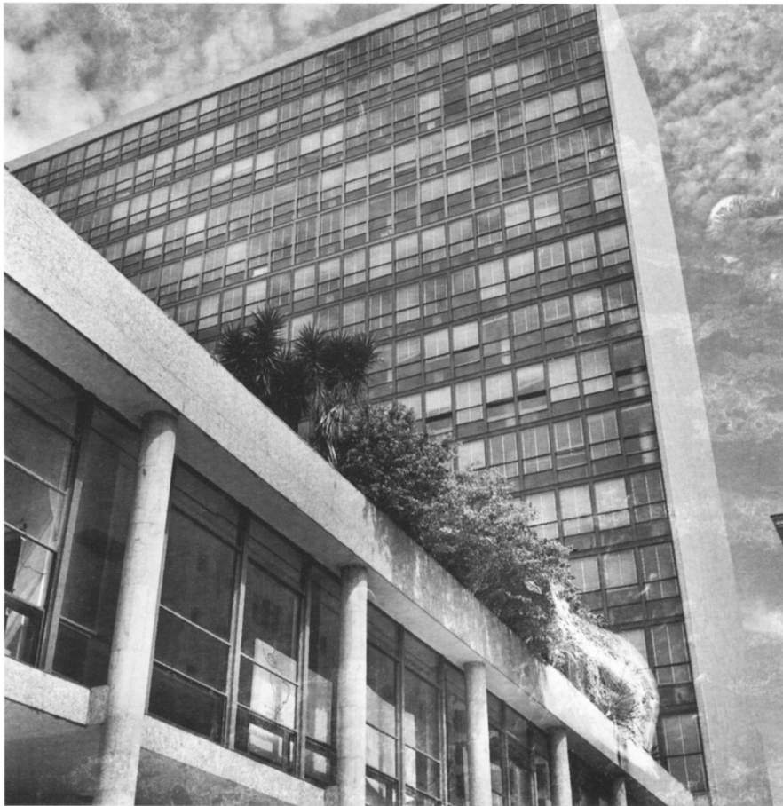
Figure 11 MES building, Rio de Janeiro, south elevation, with garden on roof of exhibition wing (foreground). Photograph by Marcel Gautherot, c. 1950
